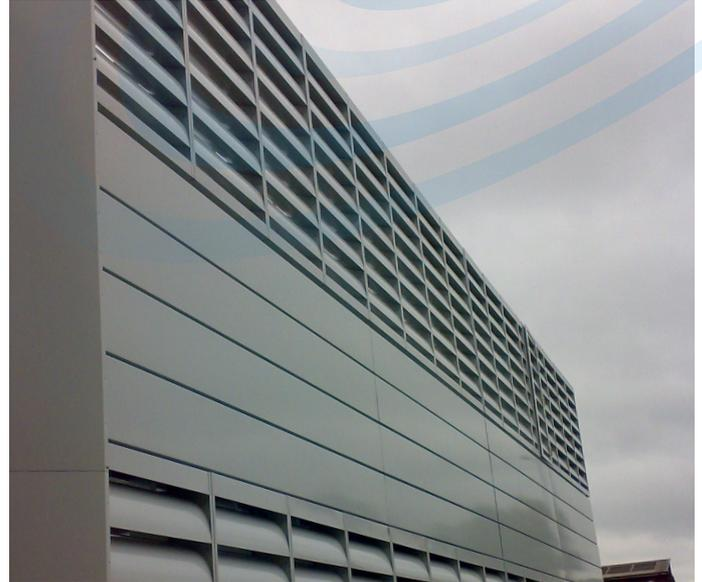
IAC designed, manufactured and installed a 50m long, 20m wide and 8m high acoustic compound to house generators at ground level and chillers on a mezzanine level. Backup power and cooling was transported into the building by means of an 18 tonne service gantry.
